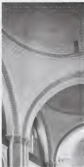
Romanesque pendentives supporting domes in the nave of the cathedral of Saint-Pierre at Angoulême, Fr., 1105–28
